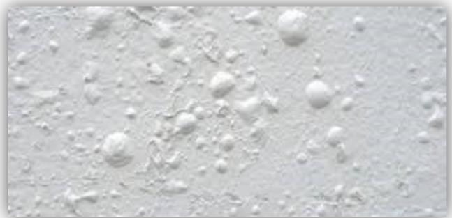
When recoating an existing court, it is important to note how many coats of surfacing already are present, and if there are many layers, to consider removing the old coats before applying a new surface. Where many layers of coating are present, each additional layer of coating reduces the permeability of the surface and increases the likelihood of bubbling.
